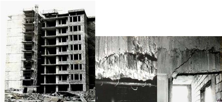
Figure 4: Block of Flats under Construction in Housing Estate “Dunav” in Svishtov (1977).
